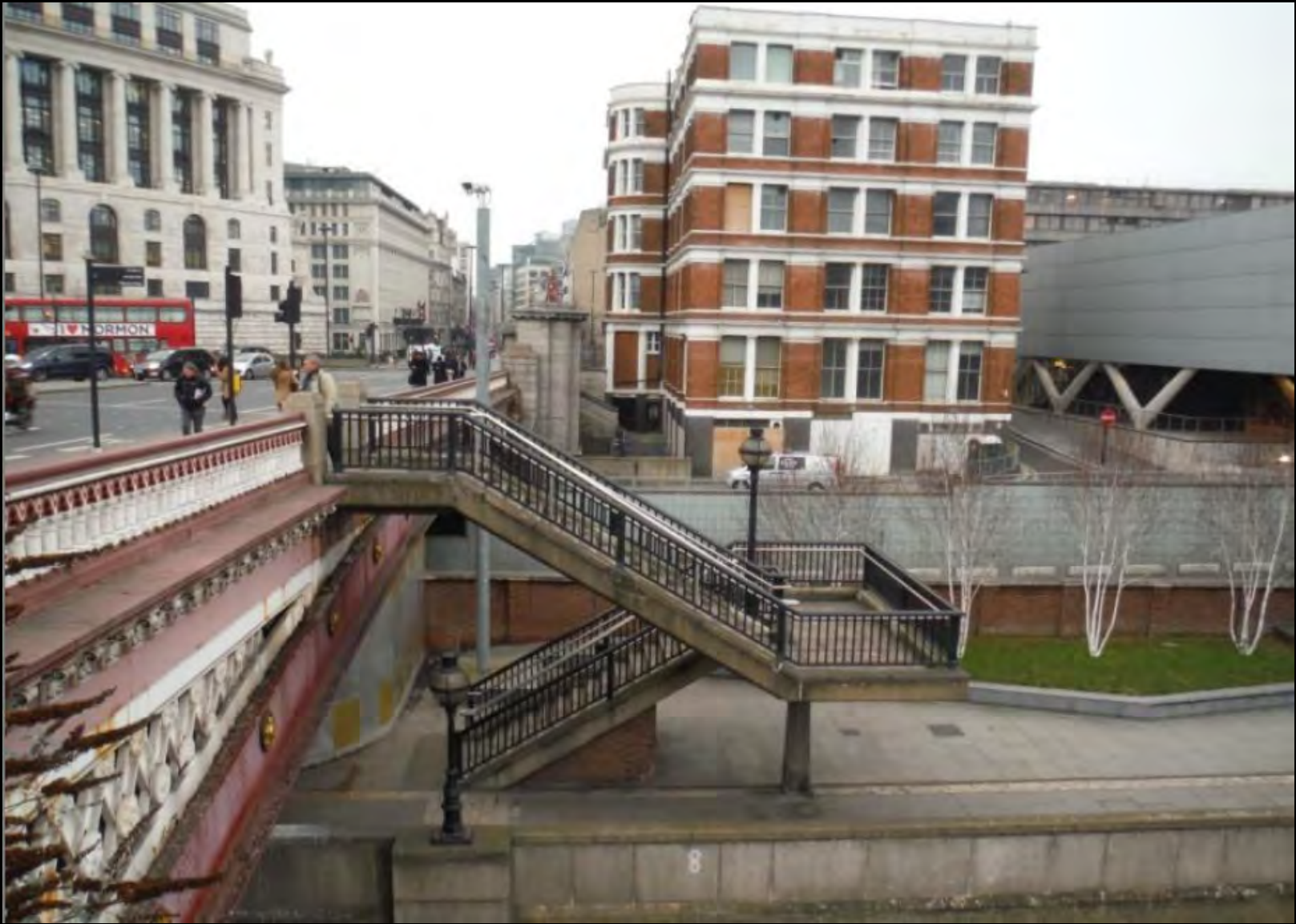
View north showing the southbound footpath on Blackfriars Bridge and the existing stairs to riverside walk
